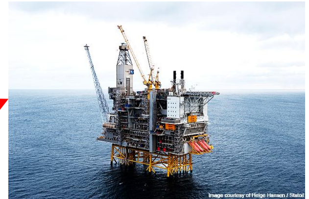
Oil & Gas Platform
