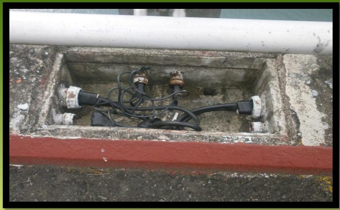
THE ABSENCE OF THE COVER FOR THE JUNCTION BOX EXPOSES THE CONDUCTORS NOT ONLY TO WATER BUT ALSO TO THE ULTRA-VIOLET (UV) RAYS OF THE SUN, CAUSING THE DETERIORATION OF THE INSULATION OF THE CONDUCTORS FASTER.
