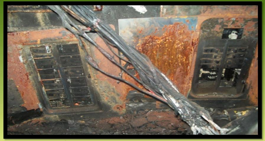
THE FLYING WIRES/CABLES WHICH INCLUDE POWER & COMMUNICA-TION LINES ARE INSTALLED TEMPORARILY.. UNTIL AN UNTOWARD INCIDENT HAPPEN AGGRAVATING MATTERS – ACCIDENTS.
