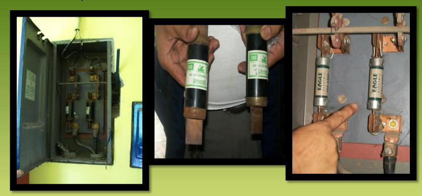
AS INSPECTED IN 2011, THE SIZE OF THIS SERVICE ENTRANCE FEEDER IS 2 – 14 SQUARE MM IN A PVC CONDUIT, SO THAT THE ALLOWABLE AMPACITY IS 70 AMPERES BUT THE PROTECTION IS 200-AMPERE FUSES!
