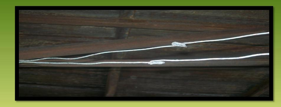
THESE INAPPROPRIATELY/POORLY SPLICED WIRES INSIDE A BADLY BURNT FLEXIBLE PVC CONDUIT. THE ELECTRICAL SUPERVISOR/FOREMAN MISSED THIS.
