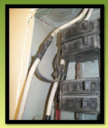
THE PLUG-IN MAINS WILL RESULT TO LOOSE CONNECTION, LOCALIZE HEATING..
