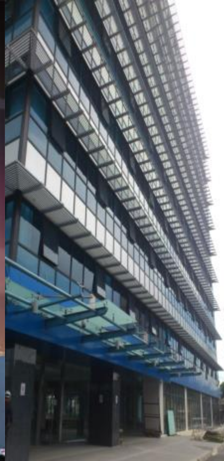
FILINVEST ALABANG BUILDING
