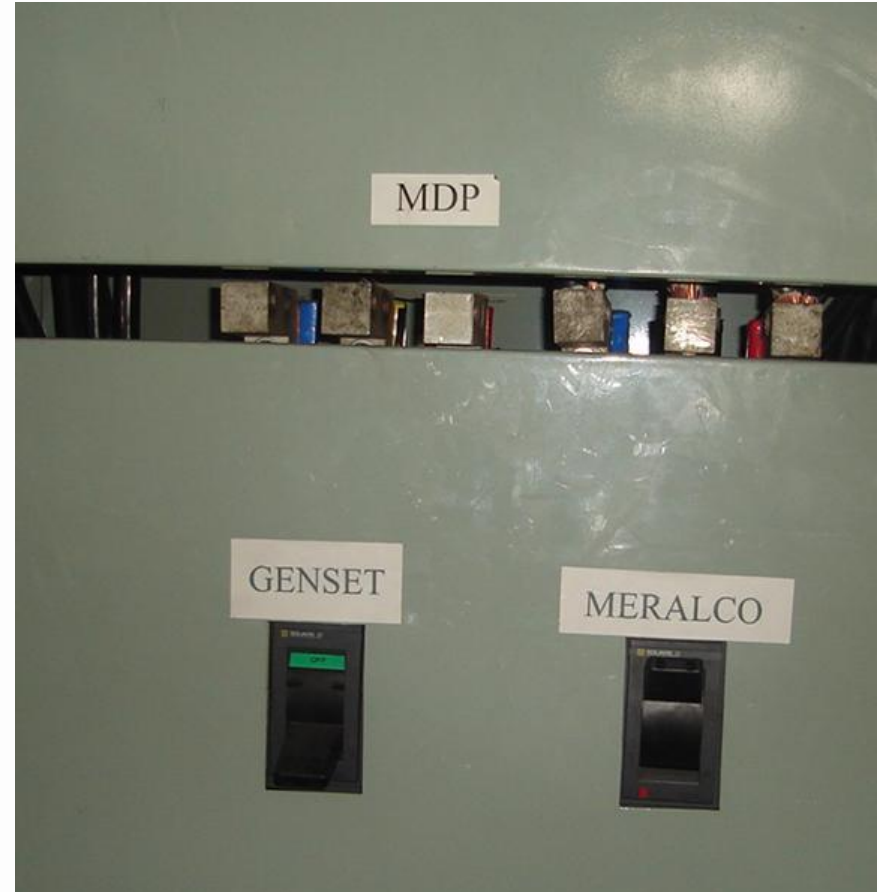
Non-automatic Transfer Switch
