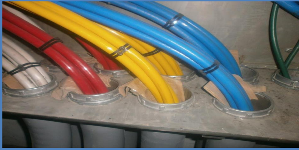
Improper cable grouping & installation
