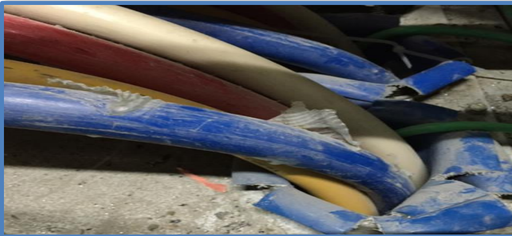
Cable damage during cable pulling and installation
