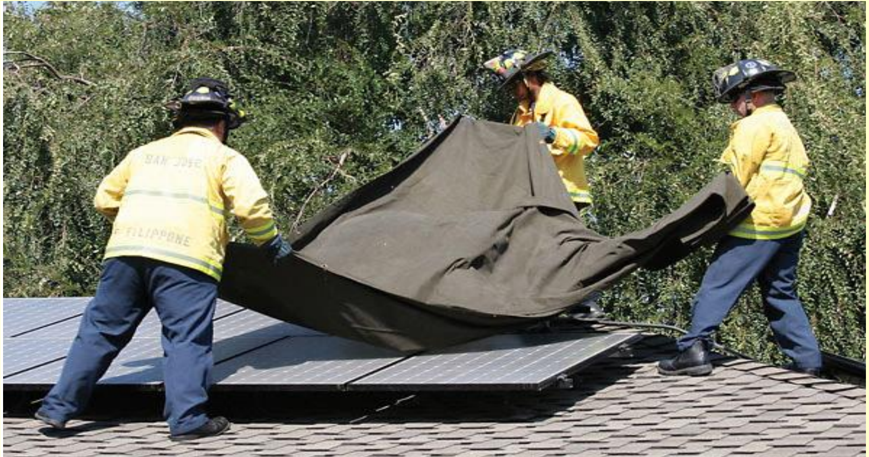
Covering panels with a heavy tarp is one approach that firefighters use to reduce voltage on a PV system (Photo courtesy of Matthew Paiss, San Jose (CA) Fire Department).
