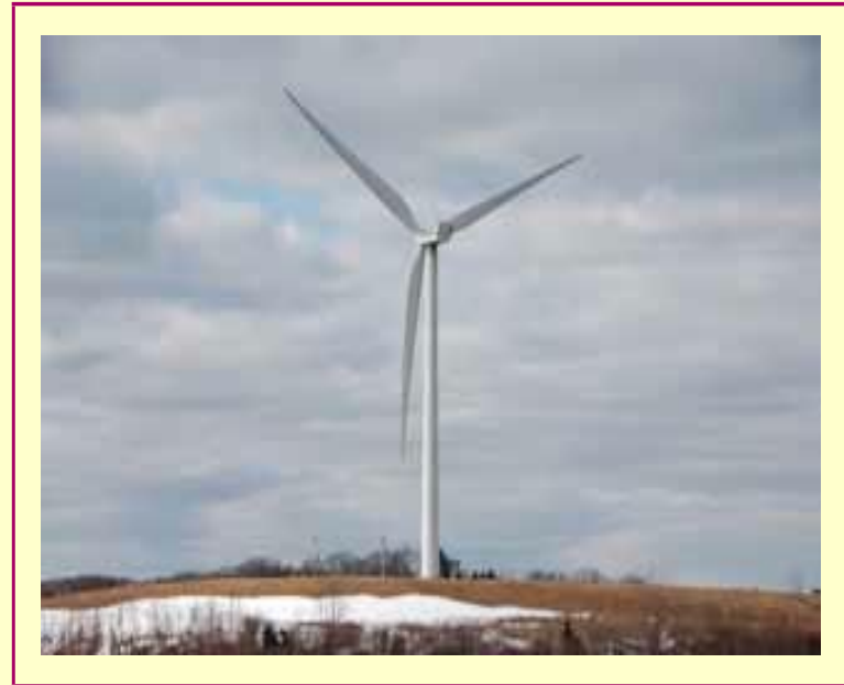
EXHIBIT 694.1 A wind electric system consisting of a single wind turbine.
