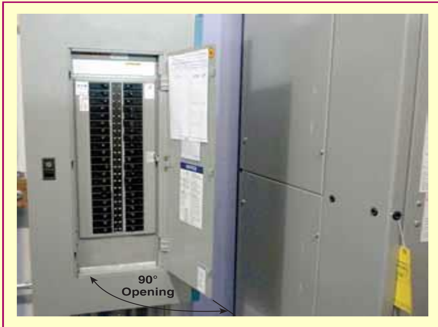
EXHIBIT 110.16 A full 90-degree opening of an equipment door in order to ensure a safe working approach.
